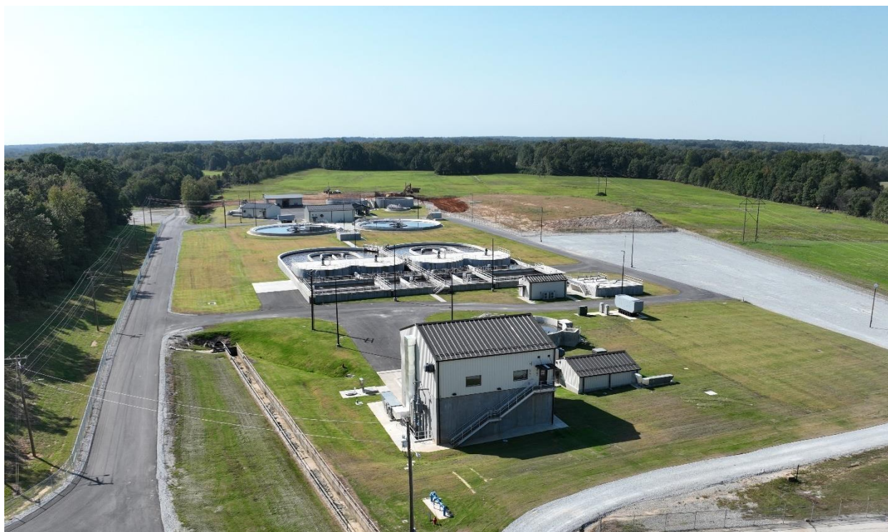
Figure 4-1: New Westside WWTP (October 2024)
